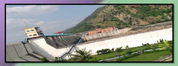
Bisalpur dam is a gravity dam on the Banas river near Deoli in Tonk district, Rajasthan, India. The dam completed in 1999 for irrigation and water supply. Various metamorphic rocks observed at the Dam site such as mica schist, quartzite, gneiss, etc. By visiting the dam site, students understood the geological features of the dam site and also the various constructional features of the Bisalpur dam.
